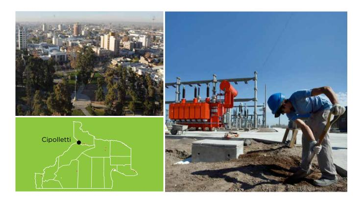
Construction of a new 132 kV Substation. The project will be built on an area of 10,000 square-meters, with two 132 KV input and output line hubs, two 132 KV bars (main and transfer), a transfer hub at 132 KV, and a transfer hub of 132/33/13.2 KV 30/30/30 MVA, 3 (three) 33 KV cells, and 6 (six) 13.2 KV cells.
