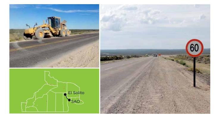
The current Route No. 2 has a length of 92 km and connects National Route No. 250 and No. 251, on the East side of the Province. The project involves drainage, underpinning and protections with waterway cleaning, granular base, irrigation of bituminous priming, hot asphalt concrete paving, underpinning and repair of shoulders, horizontal and vertical signaling.
