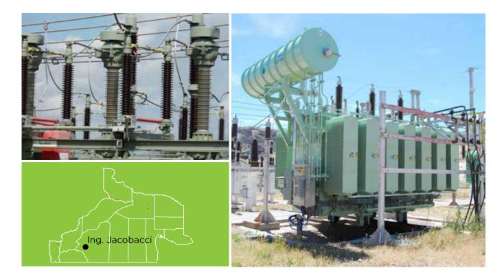
132/33/13.2 KV Substation to be built at Jacobacci Substation, with a 20 MVA transformer. A transforming hub a 132 KV/33/13.2 KV will be built and the 33 KV bar will be enlarged to enable the entrance of the new hub.
