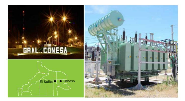
The project will involve the construction of a 132/33/13.2 KV substation at El Solito, including the installation of a 15 MVA transformer at 13.2 KV. At General Conesa, a 132/33/13.2 KV substation will be built with a 30 MVA transformer at 13.2 KV.
