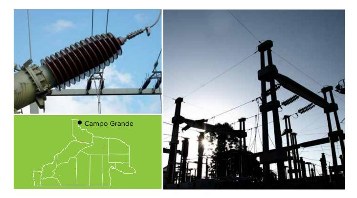
The project embraces the construction of a full Substation on a 1-hectare area, 2 (two) 132 kV line hubs, 1 (one) 132/33/13,2 kV - 15/10/15 MVA transformer with 132 and 13.2 kV equipped fields, building, etc.
